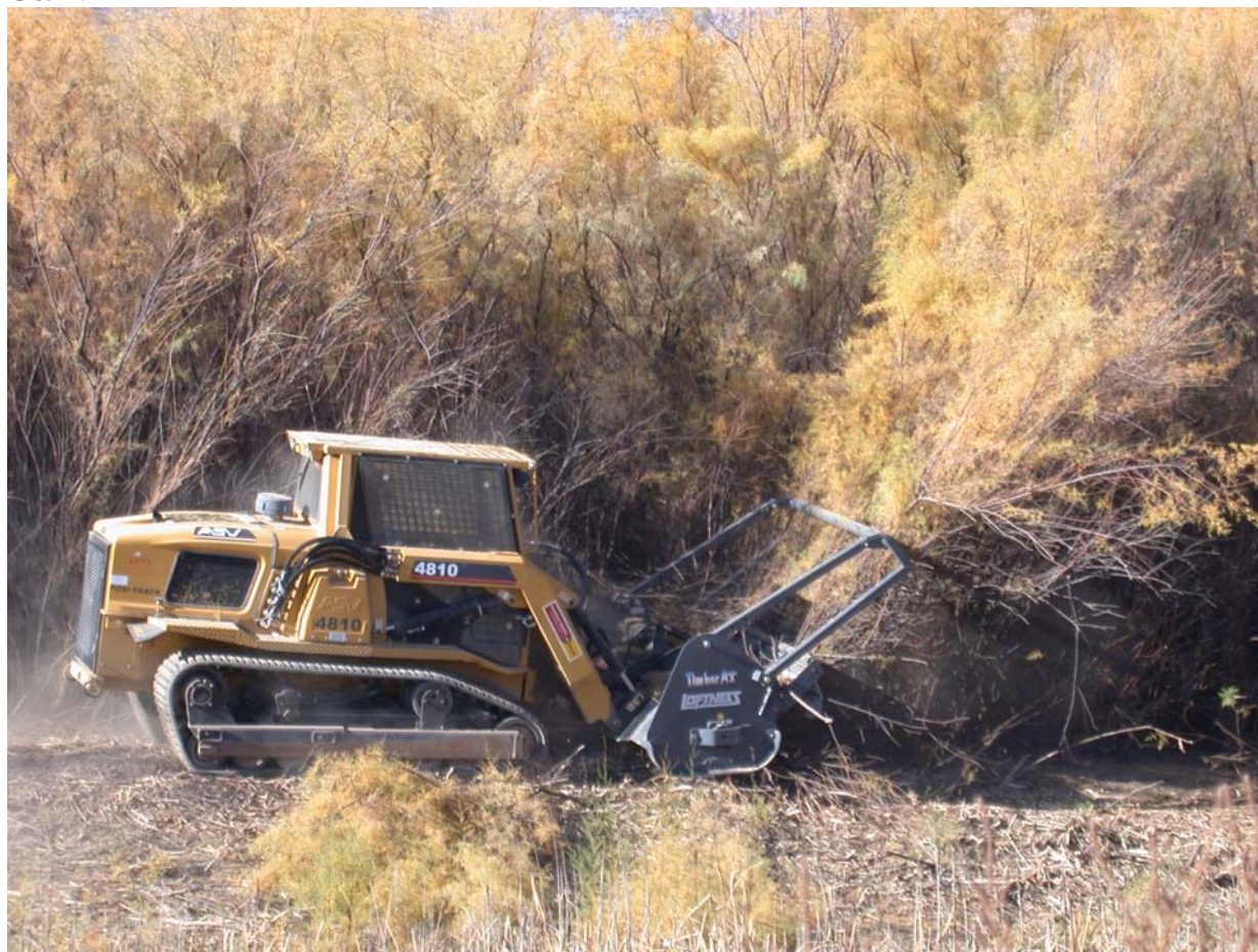
Figure 4: Medium-sized mulching equipment using a rotary drum cutting head, Moab, Utah.
